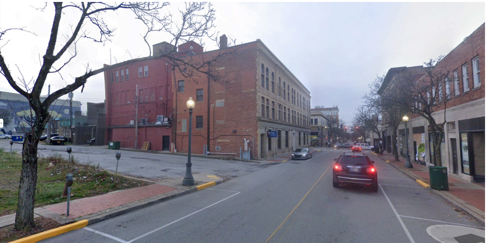
LEFT Green infrastructure can be incorporated into business district streetscape renewal and safety improvements. Individual property owners, like the one on the right, are planning for stormwater improvements.
