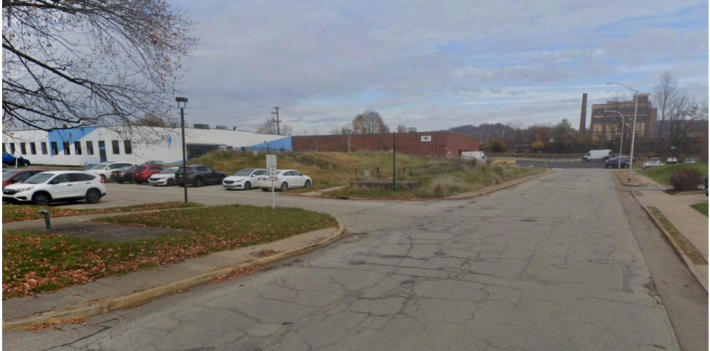
LEFT Trenton Avenue is a connector to the residential areas south of Penn Avenue. PRT has examined the possibility of a below grade crossing of the railroad and busway, which would be at the location of a historic stream.
