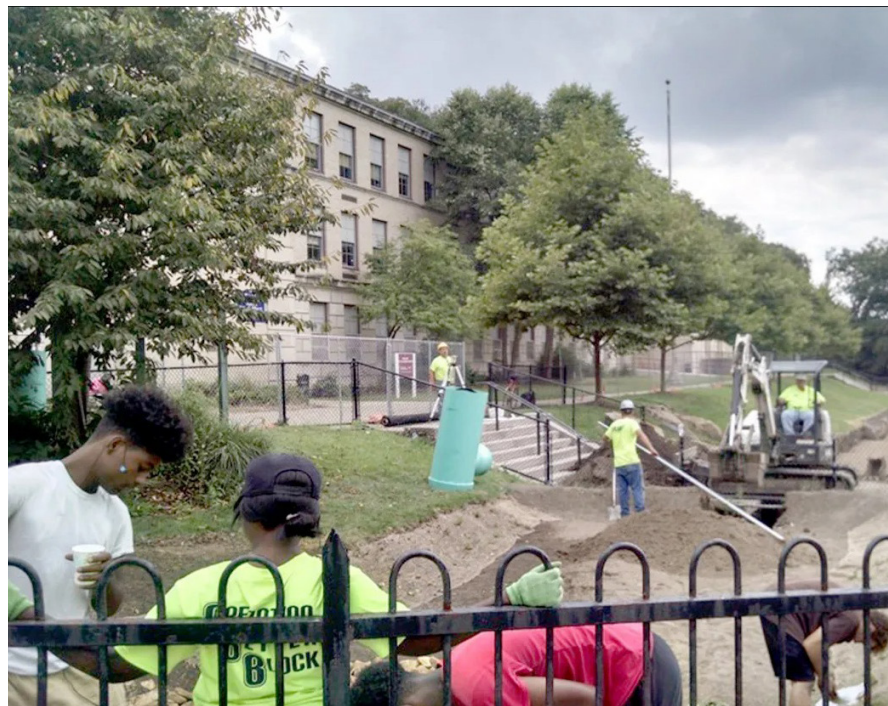
RIGHT Crescent Early Childhood Center rain garden construction (UpstreamPgh)
