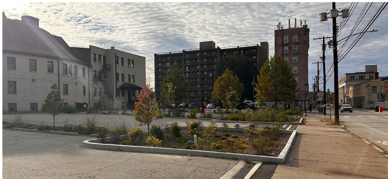
BELOW Green infrastructure was installed at Wilkinsburg’s municipal parking lot (UpstreamPgh)
